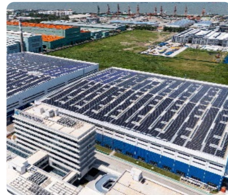
Suzhou Plant Photovoltaic Project
